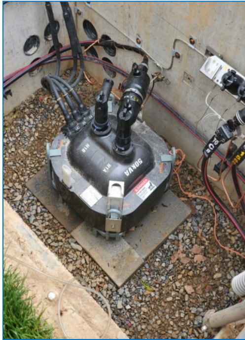
Figure 63: Example 50 KVA SIDT Transformer
