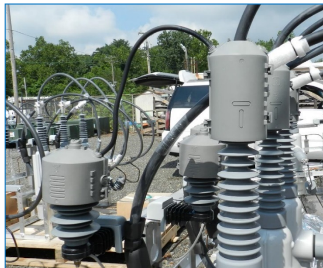
Figure 43: Example Animal Guard Installation
