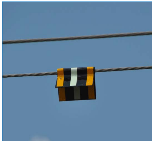
Figure 45: Bird Diverter
