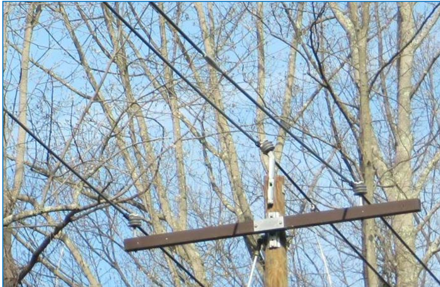
Figure 8: Example Tree Wire Installation
