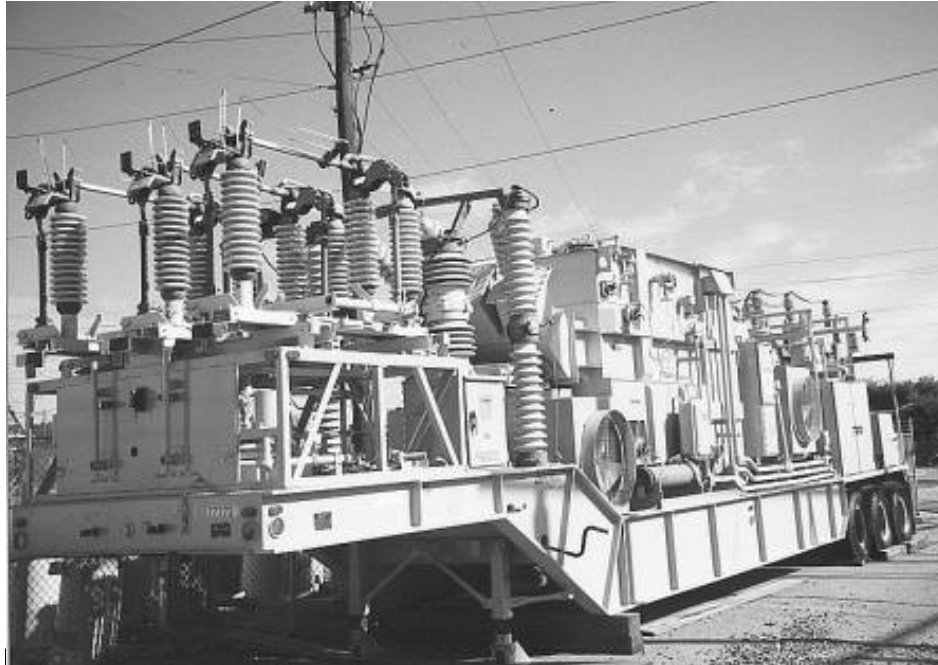
Mobile Substation
