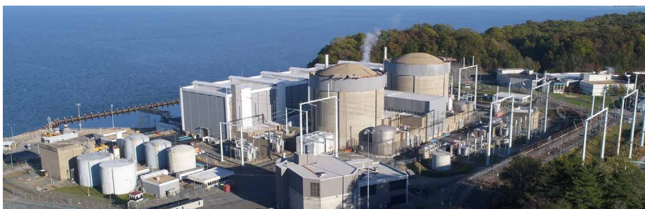
Calvert Cliffs nuclear power plant overlooking Chesapeake Bay, Lusby, Maryland.
