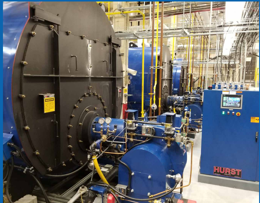
Constellation's energy efficiency project for the Department of Energy included replacing three boilers at the end of their life cycle.
