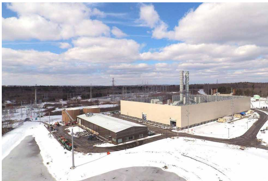
The new Medway Peaker project in Massachusetts is available to balance variable wind and solar energy resources.
