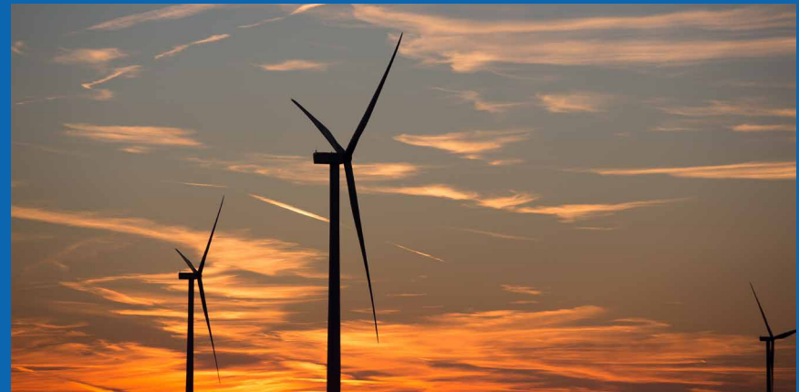
HillTopper Wind project in Logan County, Illinois.
